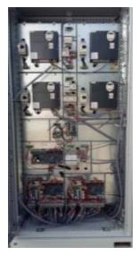
Fan drives + Pump drives + electronic boards
